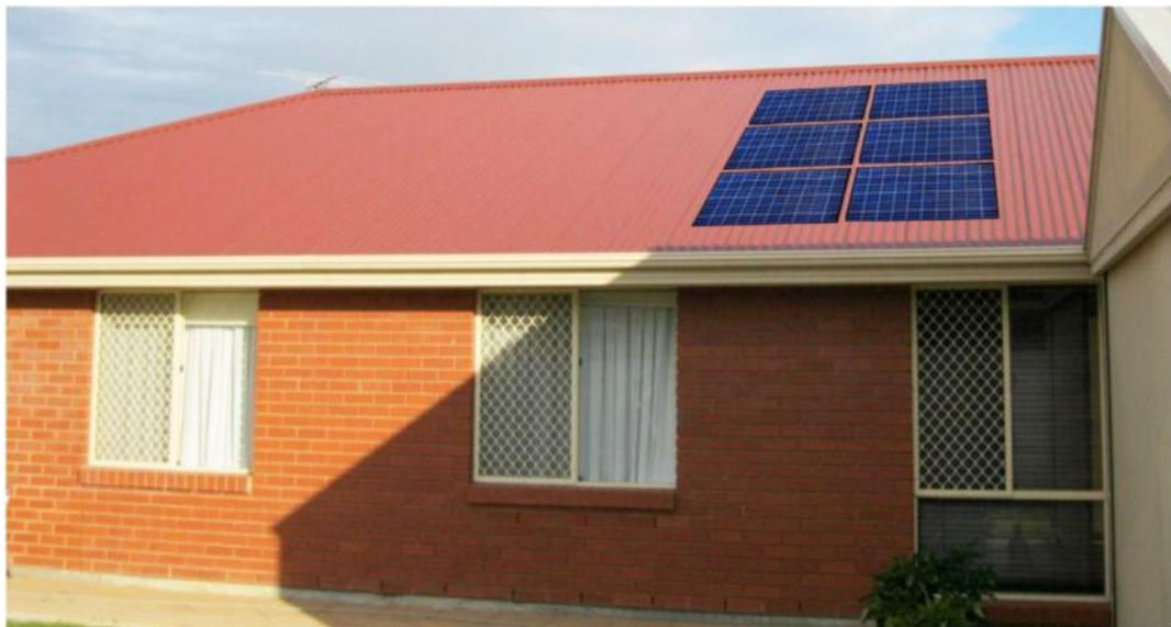
To mount the PV modules in landscape, run the SunLock rails up and down the roof, with an L-foot at each of the 5 battens. The rails may be long enough to hold four modules, filling the space completely from ridge to gutter. However, there might not be enough fixings to hold down four modules.
